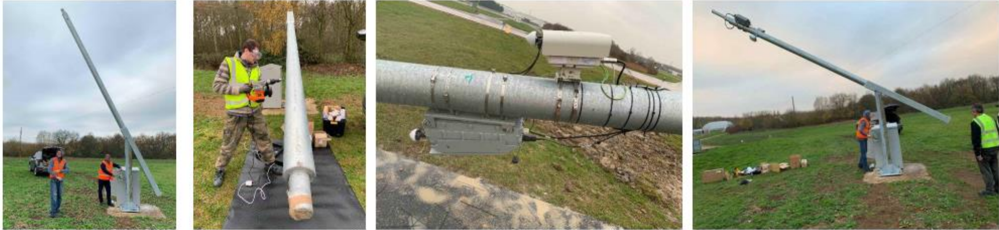
Lowering, Drilling, Equipping and Erecting Flat Area Masts
